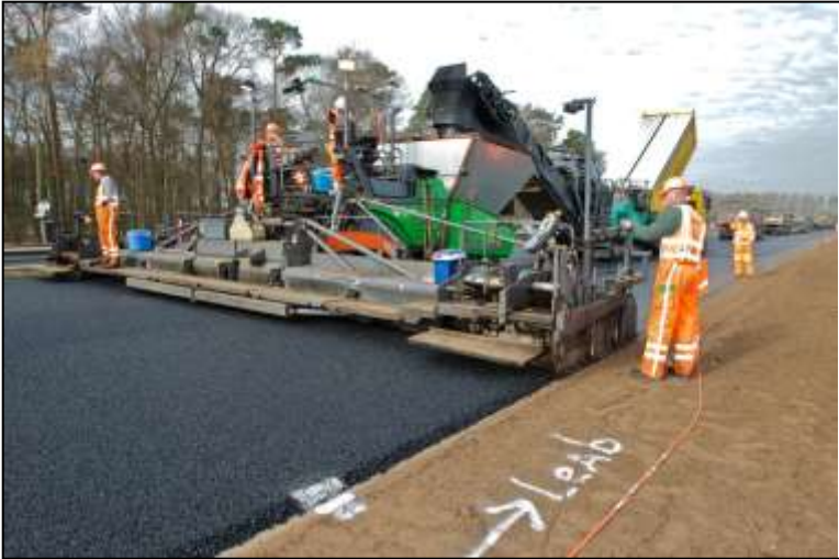
Low Energy Asphalt
