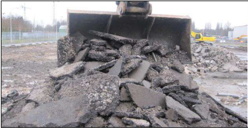
Asphalt with high % recycled materials
